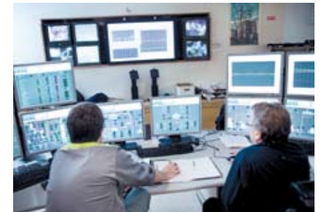
▲ Fiberline operators in the control room at Stora Enso’s Skutskär Mill.
