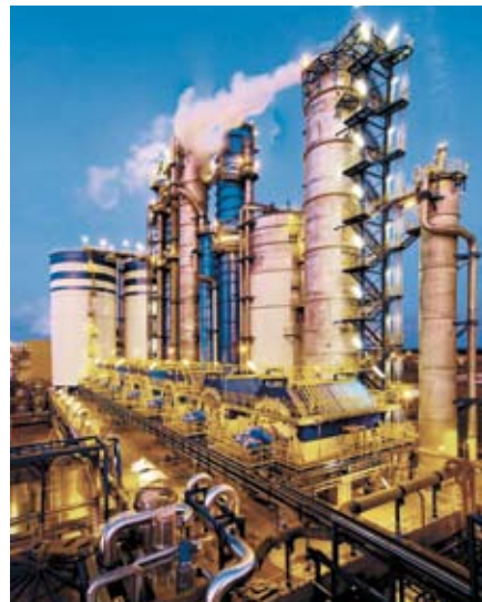
▲ Two views of the ANDRITZ fiberline at Três Lagoas. Left: The single-vessel continuous digester is currently ANDRITZ's largest. Right: Large DD washers are employed for washing and bleaching.
