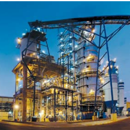
▲ Two views of the ANDRITZ fiberline at Três Lagoas. Left: The single-vessel continuous digester is currently ANDRITZ's largest. Right: Large DD washers are employed for washing and bleaching.
