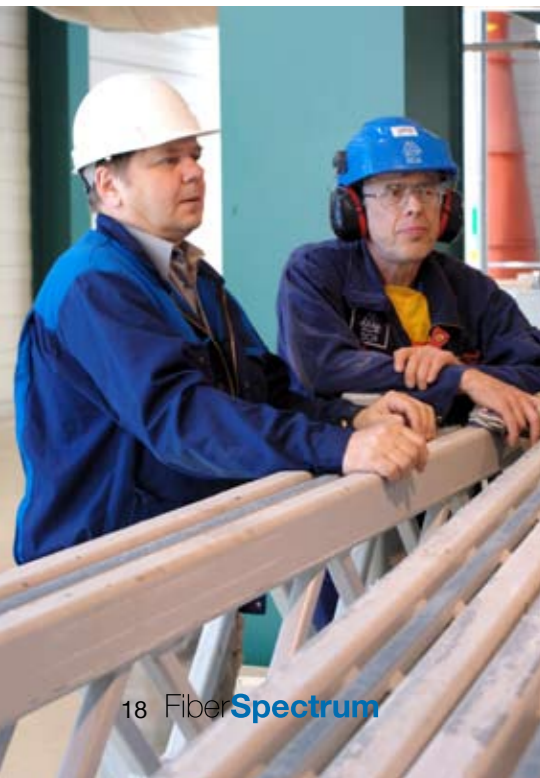
▼ Lars-Gunnar Magnusson, Andritz Service Manager (left), with Lars Åke Larson, Boiler Operator, inside the new Andritz recovery boiler.
