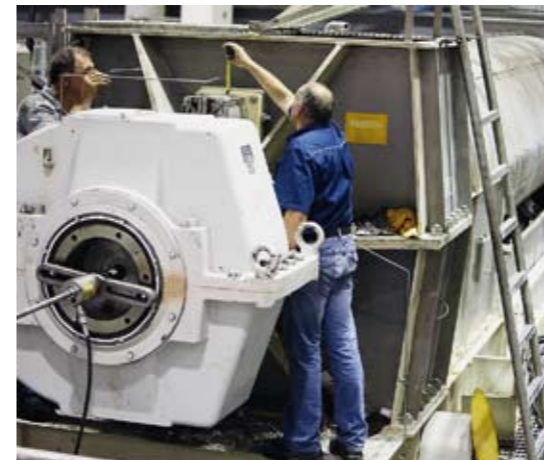
▲ Gottfried Prettenthaler (left) and Hans-Peter Ritter, both Andritz Erection Supervisors, check the piping of the pneumatic back-pressure device on screw press #5.
