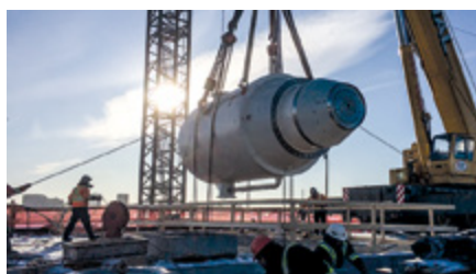
Installation de la turbine Bulbe
