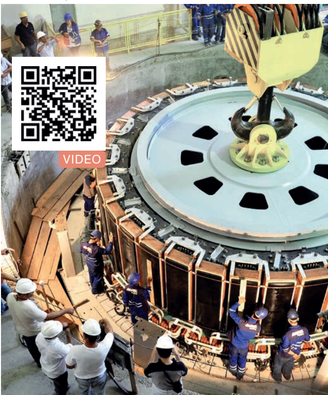
Installation of generator at HPP Mauá
