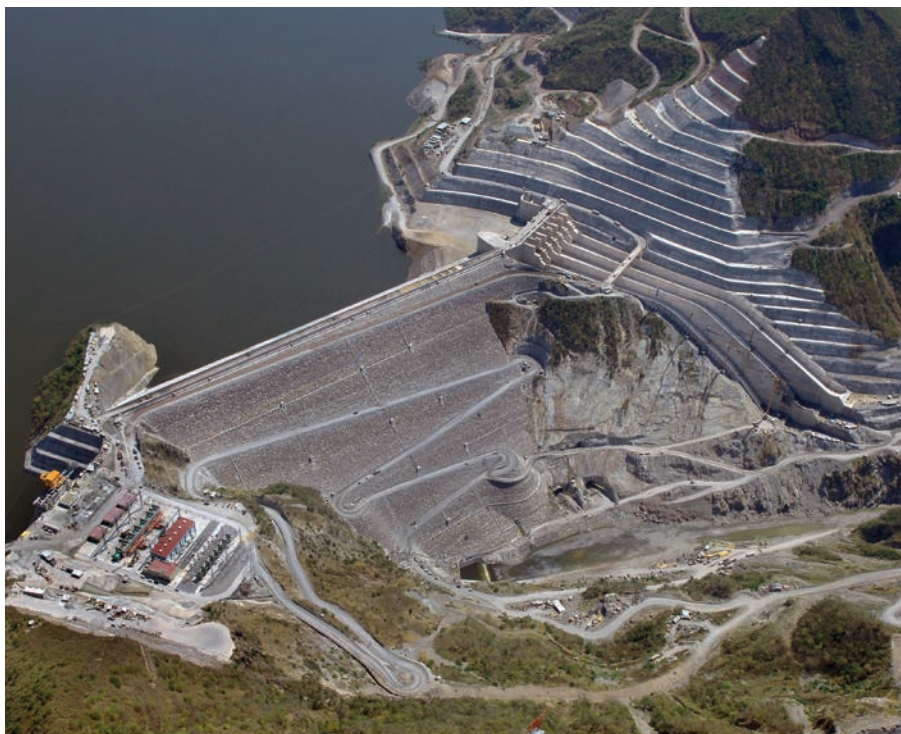
Reservoir and power house of HPP La Yesca
