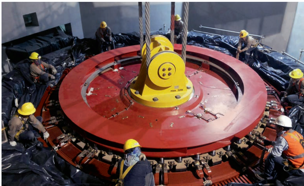
Installation works at HPP Cerro del Águila
